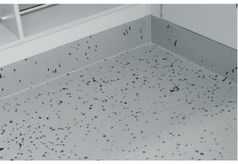
■ FLOOR COVERING: Floor spray covering, with edges extending up on side walls – non-slip and easy to clean.
